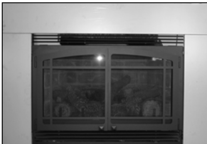
Completed Shroud Installation
