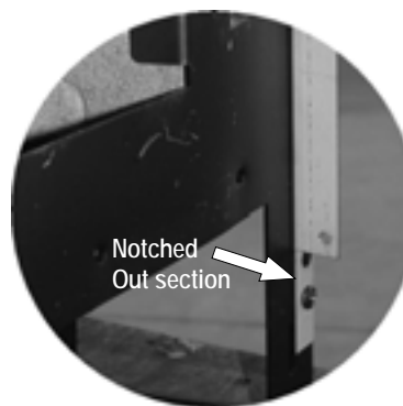
Figure H-5 - Note flange orientation
